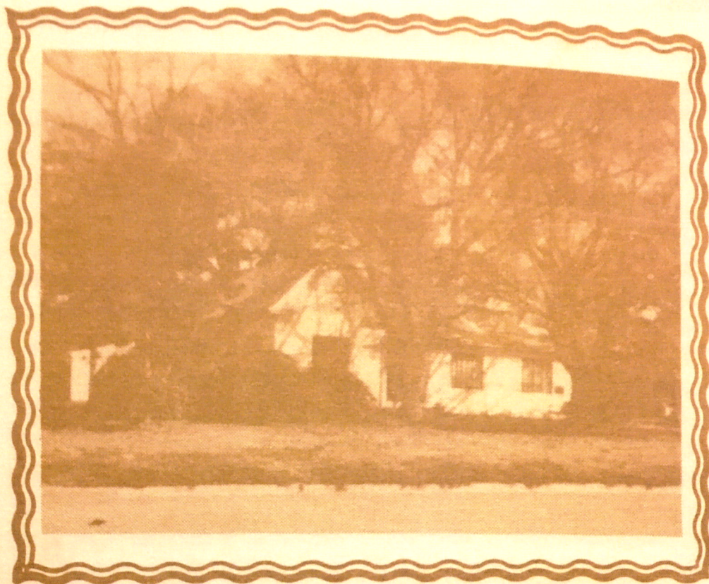
THE HAEDGE HOME, built about 1892.
